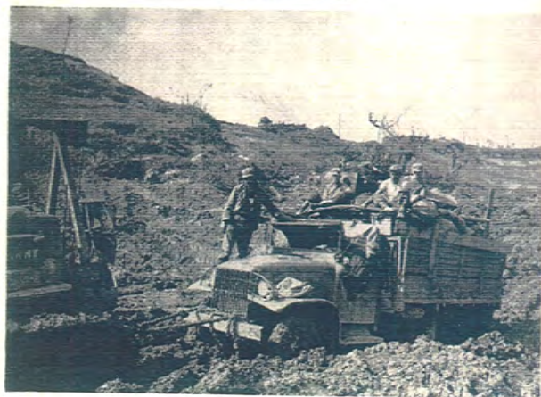
Top: A lineman exposes himself to enemy fire as he repairs telephone wires. Bottom: A bulldozer of the 302d Engineer Combat Battalion pulls a truck through a bad stretch of road north of Shuri.
